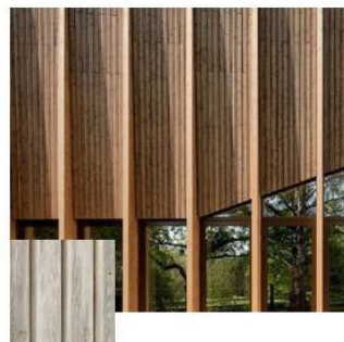
TIMBER CLADDING Preferred: Thermowood or similar
