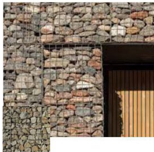
GABION 4mm gauge welded mesh cage with stone aggregate sourced from local quarry.
